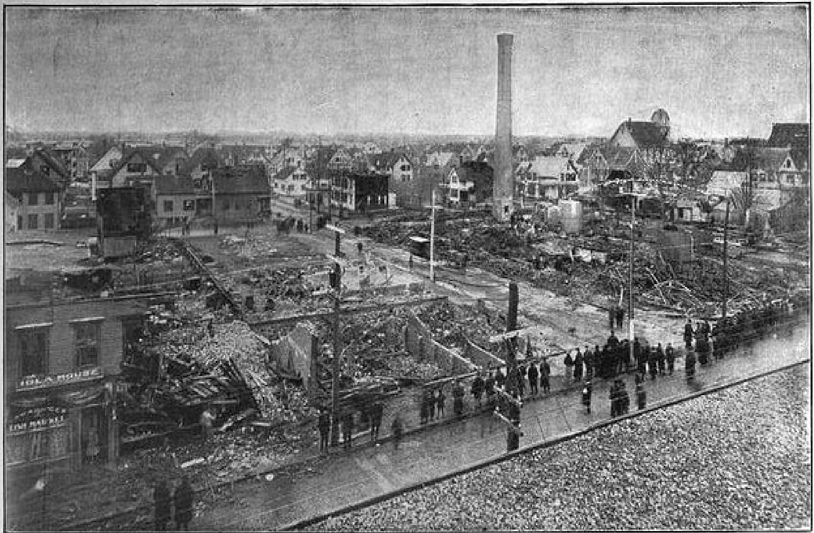
AFTER THE EXPLOSION AND FIRE. Looking west. Smokestack and ruins of Grover Factory at right; Dahlborg Block at left; ruined dwellings in background. Curved white line shows path of boiler from base of smokestack to house of Miss Pratt, where it lodged.
