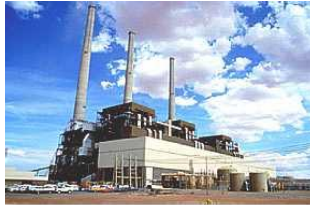
Navajo Generating Station
