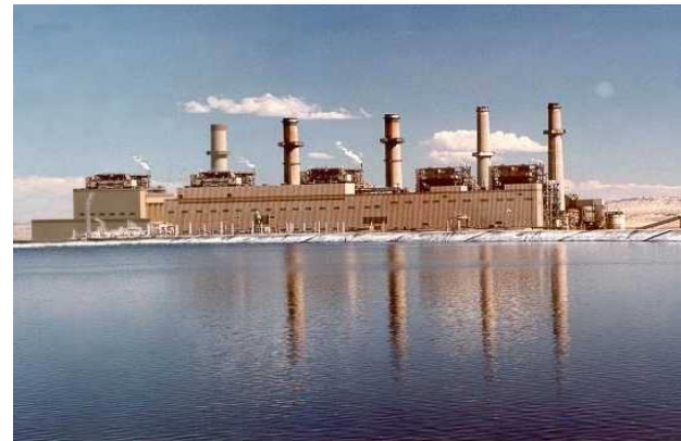
San Juan Generating Station
